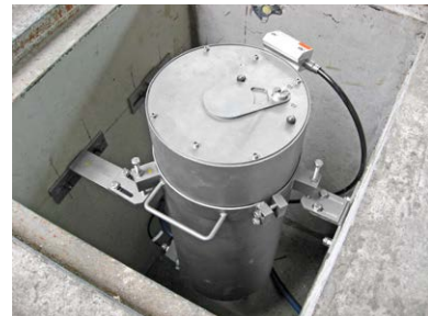
Protective housing with purge collar, cooling and pneumatically driven protective cover
