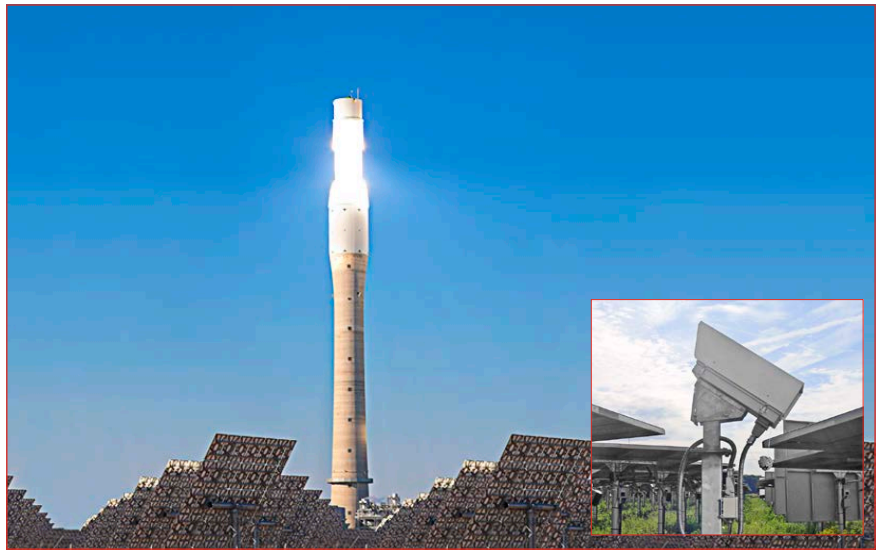
Solar tower power plant – Monitoring the optimum heat distribution using infrared cameras from InfraTec
