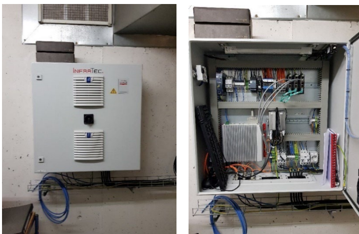
Fig. 5: WASTE-SCAN 4.0 control and evaluation unit
