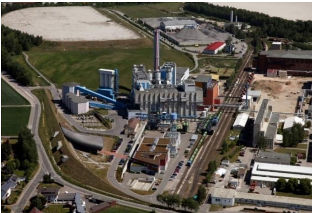
Fig. 1: Overall view of the ZMS Schwandorf WtE plant
