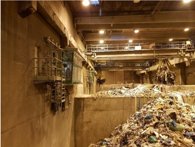
Fig. 2: Bunker view with crane cockpit on the left
